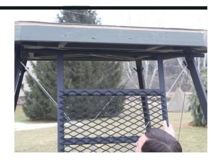
18 Fasten the nut onto the end of the platform. This keeps the platform in place.
