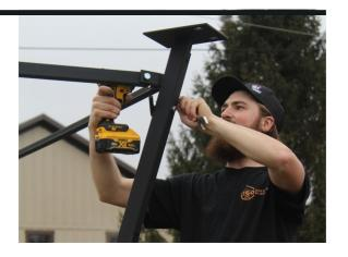
Install the diagonal cables between the legs of the blinds and hand tighten.
