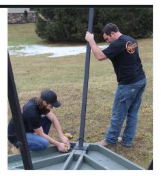
The edge of the leg bracket should be even with the edge of the 4x4 in the bottom of the blind floor.
