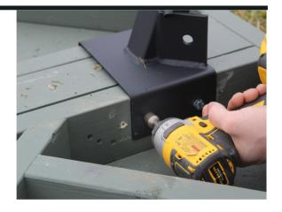
Note all 4 legs installed. IMPORTANT!! Make sure the legs with the extra bracket for the ladder platform get installed on the "Door" side of the floor as shown in the picture!
