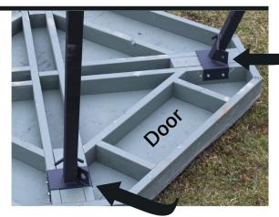
Install horizontal braces as shown.
